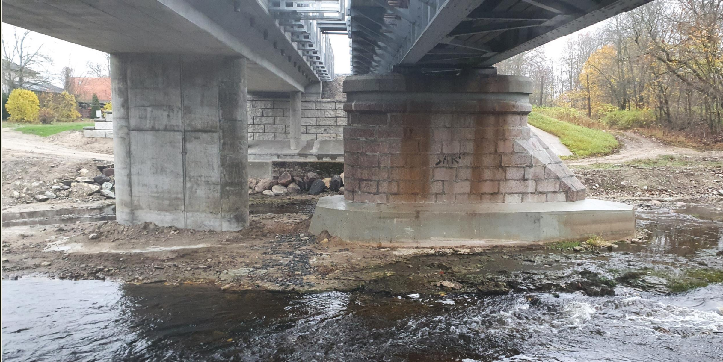
Under railway bridges, October 2022
