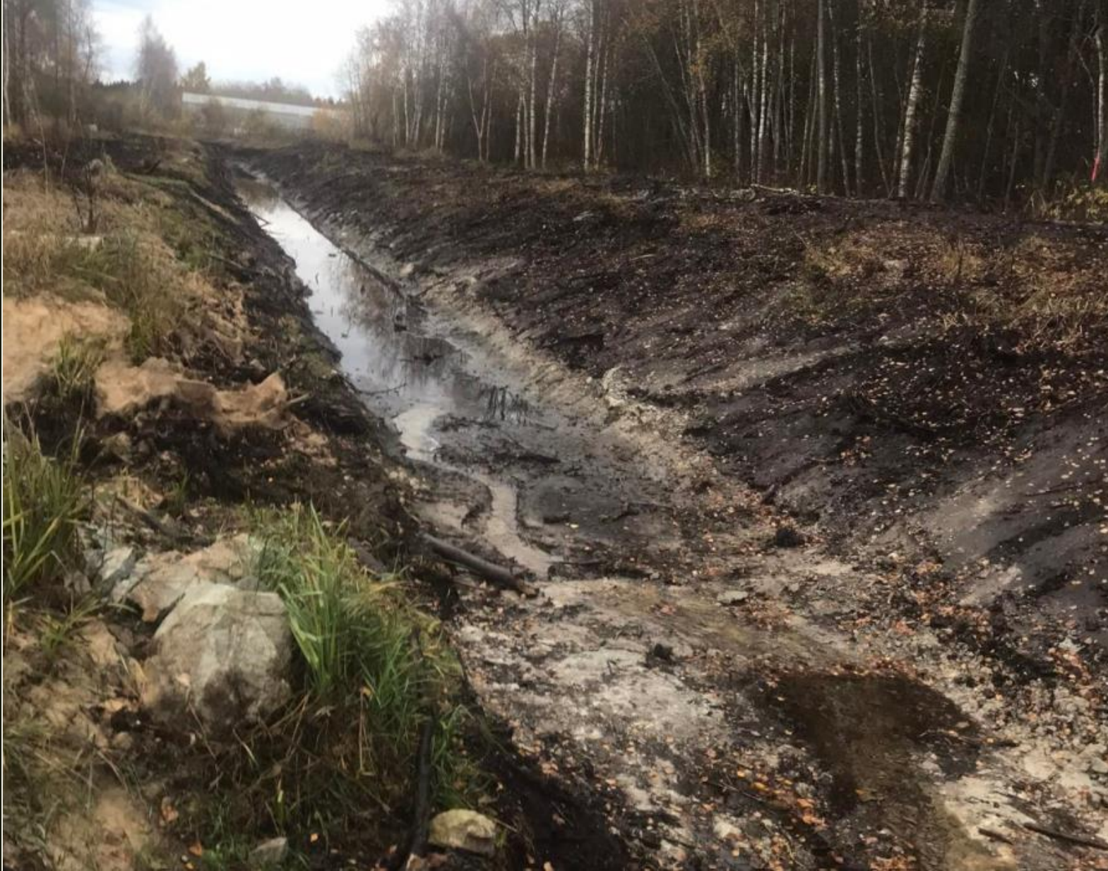
Renewed ditches, October 2022
