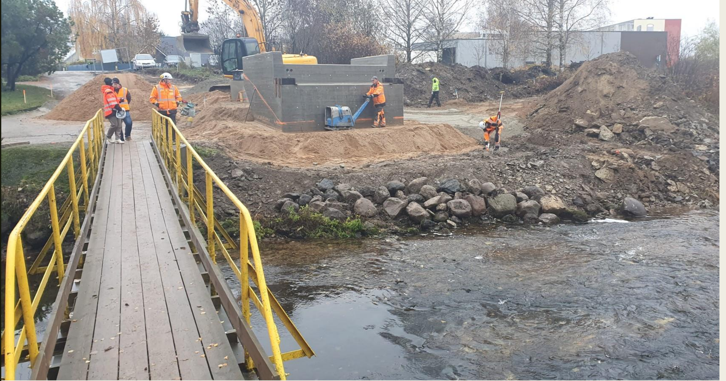
New pedestrian bridge Under construction, November 2022
