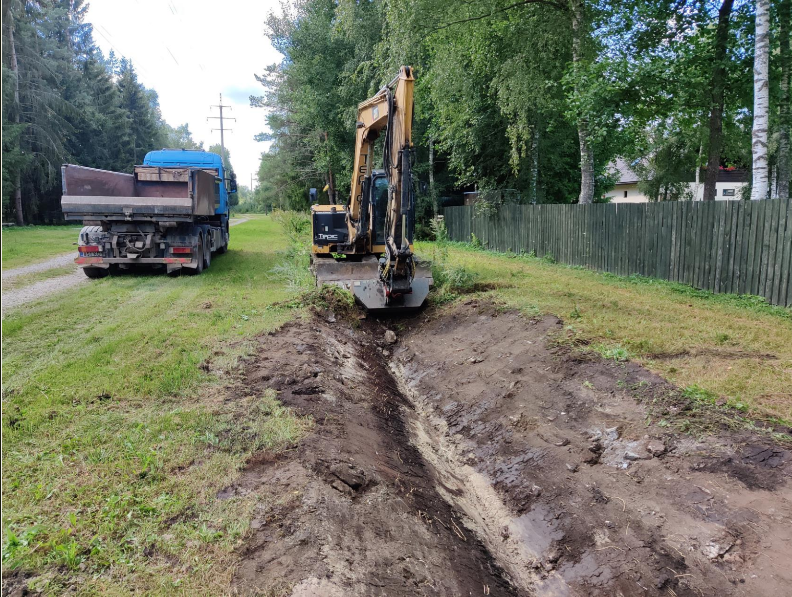
Renewed ditch in Southern Keila, August 2022
